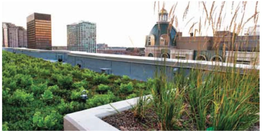
An extensive green roof covers part of The Mather's south building. This roof, which requires minimal care, consists of indigenous species of mostly sedum plants and native grasses. It is among the sustainable features contributing to the building's recent LEED Gold certification. Image courtesy of Mather LifeWays
